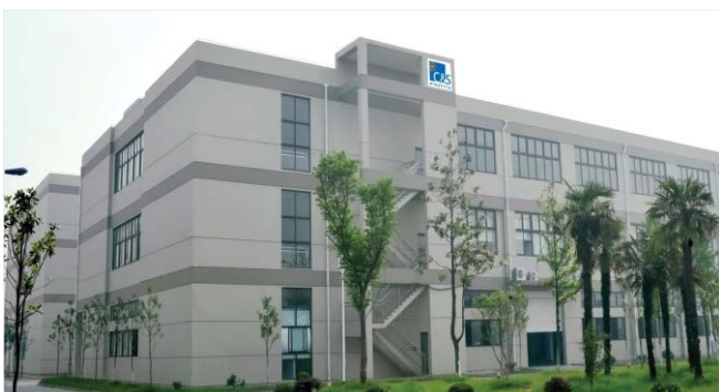
C&S (Nantong) Electric Plant - CHINA
