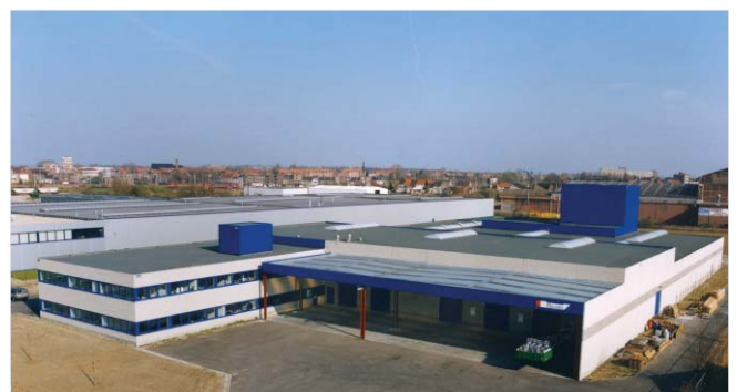
C&S+Eta-com Plant - BELGIUM
